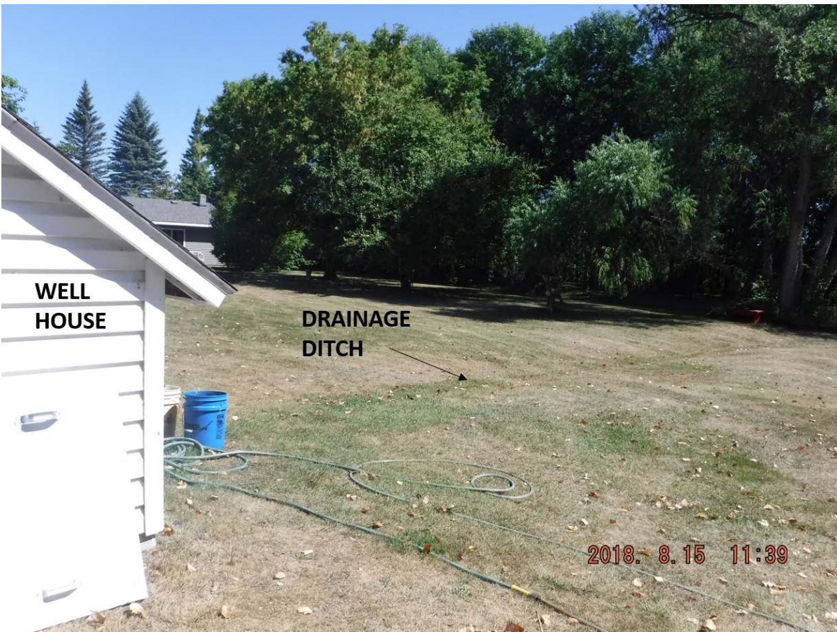
Figure 3. Photograph of the Lessard overflow drainage ditch.
